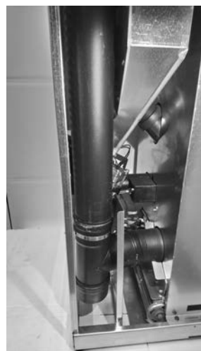
Fig. 56 - Raccordement "T"
