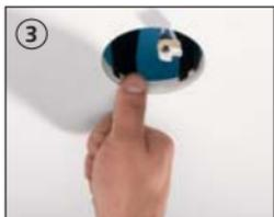
Push the retaining spikes into the plasterboard to prevent subsequent shifting.
