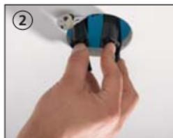
The 4 flexible mounting clips will lock easily into required position.
